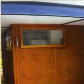
Plywood sheeting inside for warmth.
